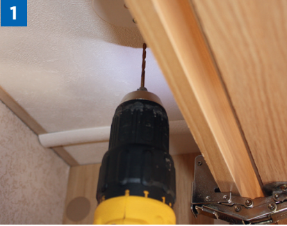
1 Drill the hole for the cable
