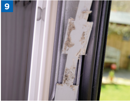
Damaged PVC strip is then removed via the widened section of the track
