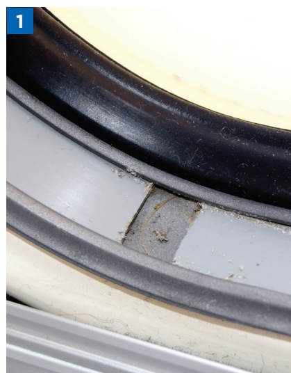
A split in this PVC strip rendered the left-hand window catch inoperative
