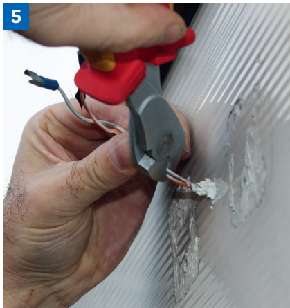
Cutting and insulating the old wires
