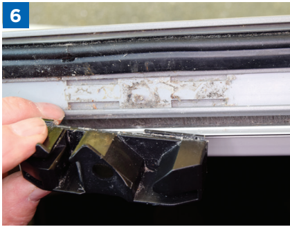
Block removed, showing four recesses driving strip when catch is operated
