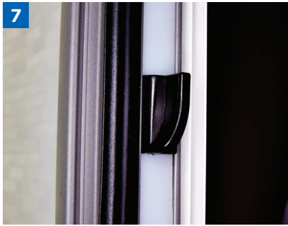
To remove side catches, push inwards with screwdriver then pivot from runner
