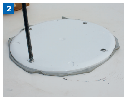
Secure new mount to roof using old holes
