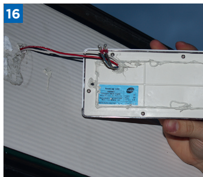
16 Sealant on back of the replacement unit
