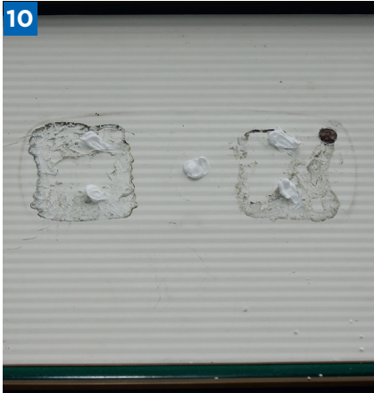
Sealing the holes from the old light unit
