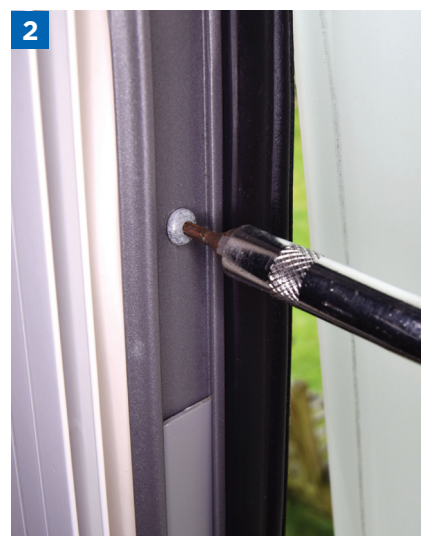
Remove the end-stop screw from the left-hand side of the window frame
