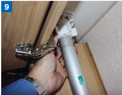
Attach and secure the locking collar
