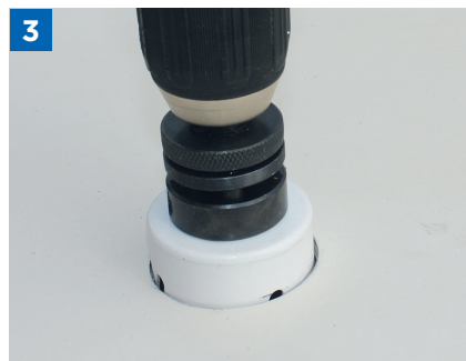
Carefully cut the 50mm hole
