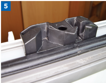
Using two screwdrivers, push to release lugs, then pivot block out from runner
