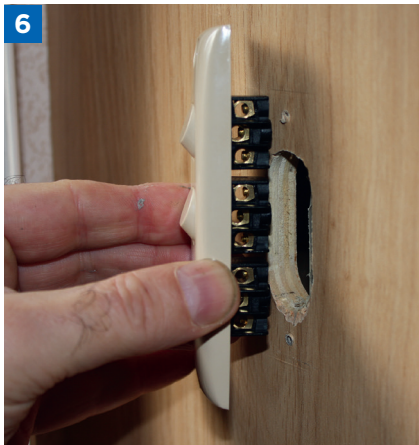
The new switch and the old hole
