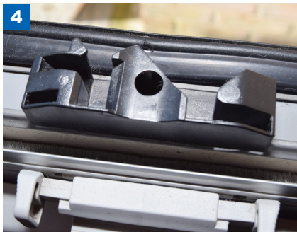
The central sliding block is now ready to be removed from the window frame
