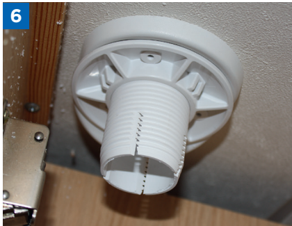
Secure tapered washer and locking plate
