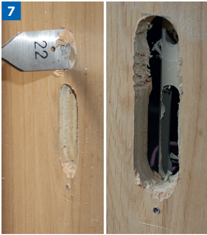
Using a 22mm wood bit to open up hole
