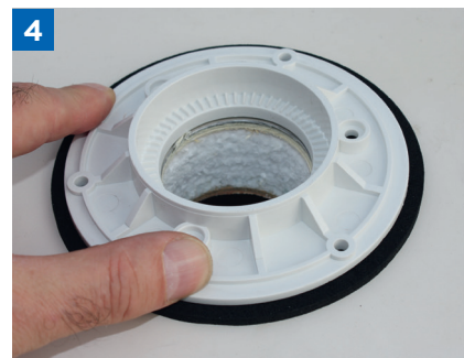
Place mounting plate over the hole
