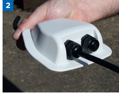
2 Feed cable via roof leadthrough housing
