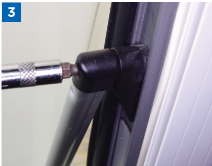
Next, remove the window stay-bracket from the right-hand side of the frame
