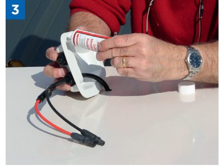
3 Apply bead of adhesive to housing
