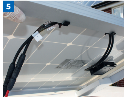
5 Secure cables with clips/ties supplied
